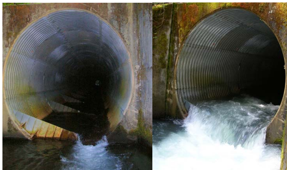
Figure XII-39. With increasing flow the water surface in the baffled culvert rises more than the tailwater pool, and a small hydraulic drop becomes much larger. The drop at high flow also causes water to drawdown and acceleration as flow approaches the culvert outlet, potentially creating a velocity barrier.
