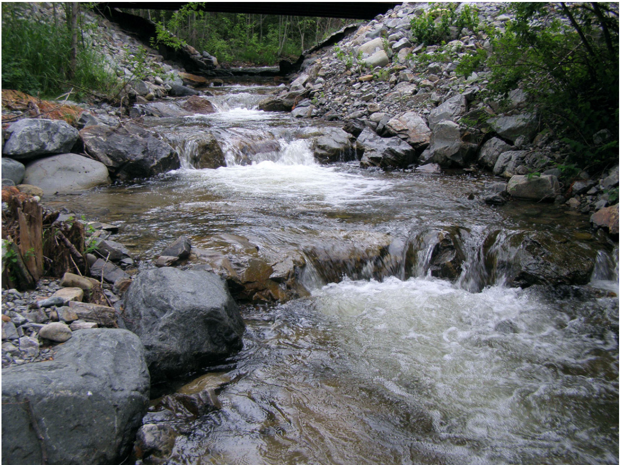
Figure XII-32. Arch-shaped rock weirs produce diverse hydraulics across the crest while concentrating flow towards the channel center. Photo courtesy of Rob Sampson.
