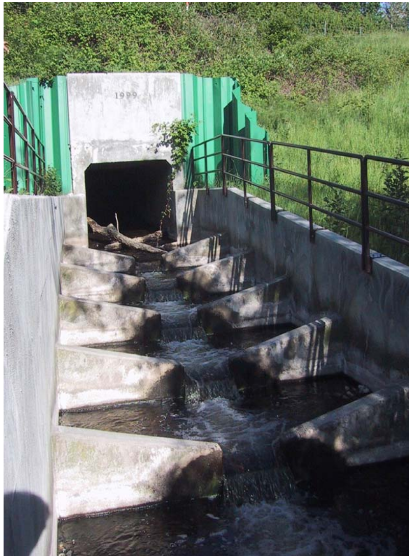
Figure XII-48. Fisher Creek pool-and-chute fishway at low flow.
