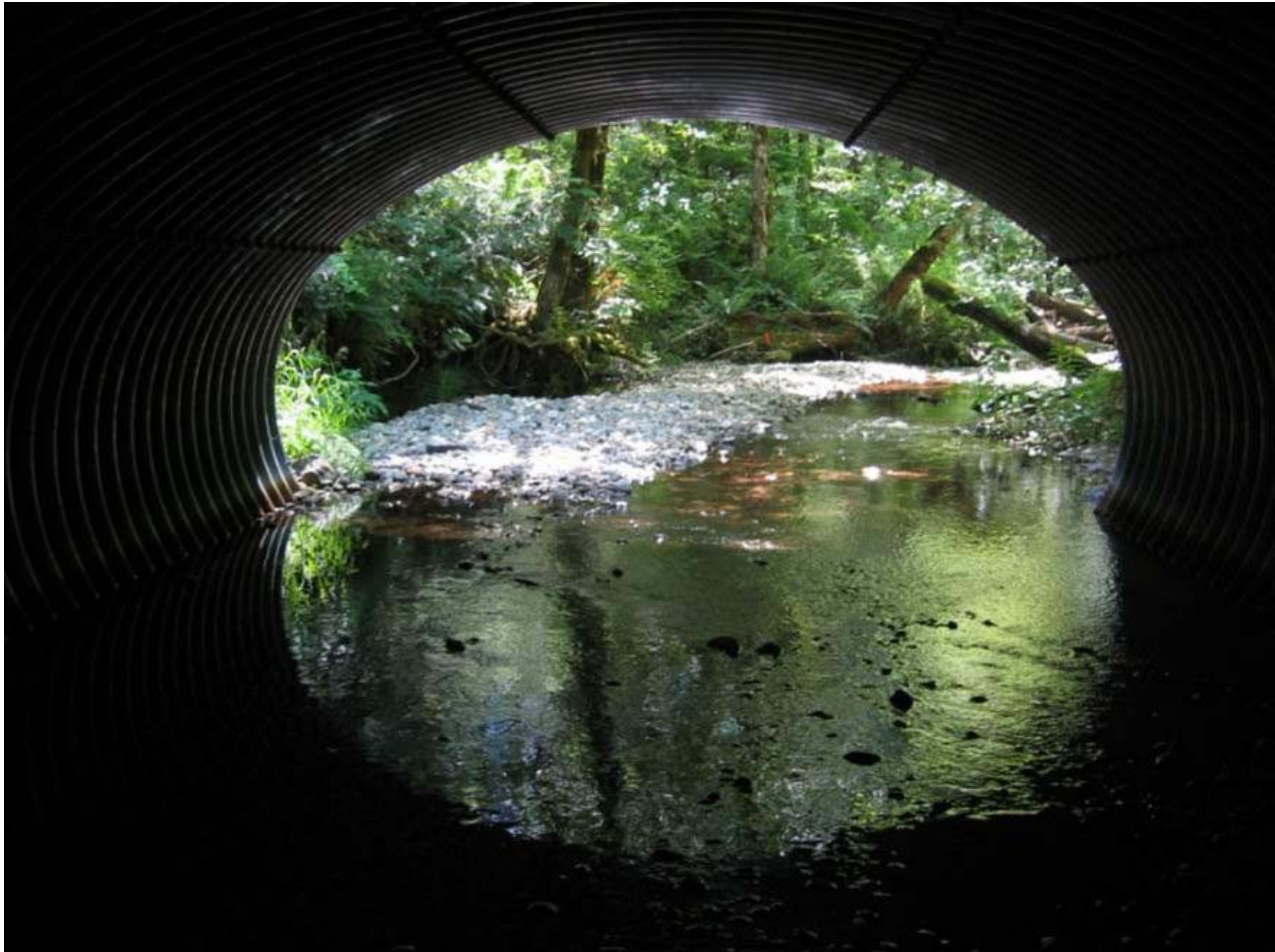
Figure XII-13. Deep Creek. Comparison of diverse bed created by woody vegetation that disrupts the flow and a flat shallow-flow bed within the culvert (Photo: Kozmo Bates).
