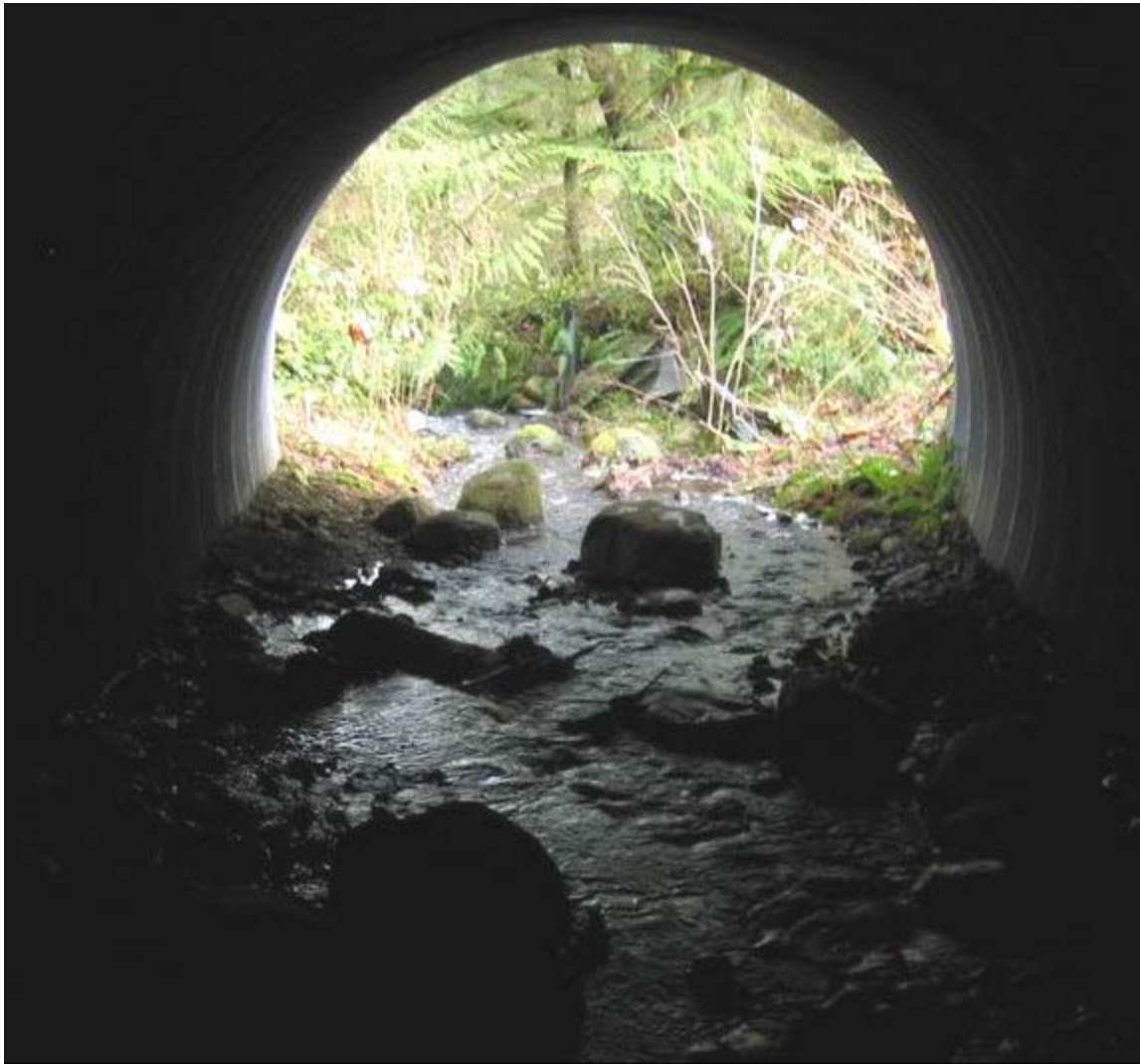
Figure XII-15. Stream simulation channel in Stossel Creek culvert with natural shape, dimensions and key features.
