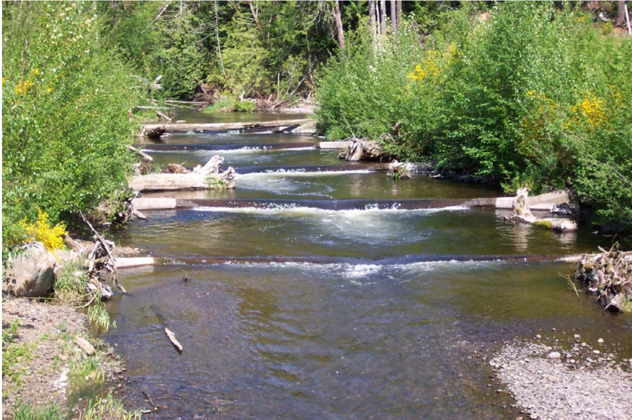
Figure XII-34. Goldsborough Dam Removal Project. An example of V-shaped rigid weirs.
