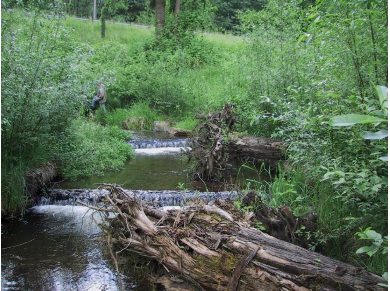
Figure XII-35. Schoolyard Creek bank protection with large wood. No riprap was used on the project. Constructed 2000.
