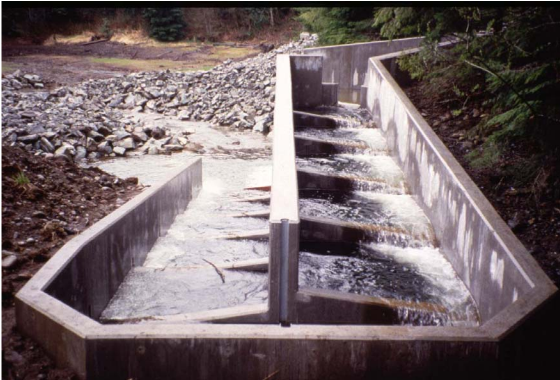
Figure XII-46. Little Park Creek fishway design for juvenile salmonid passage. Baker Reservoir, WA.
