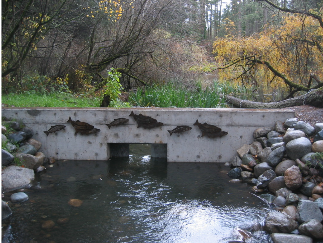
Figure XII-54. Flow control structure, Spanaway Creek bypass channel.
