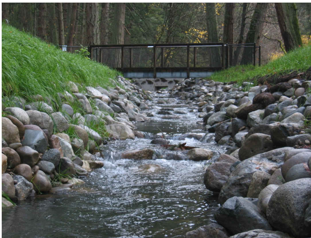
Figure XII-53. Spanaway Creek bypass roughened channel.
