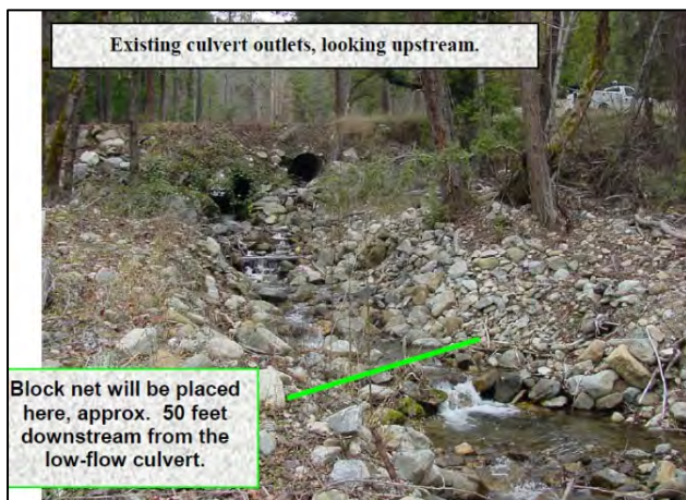
(C) CULVERT OUTLET
