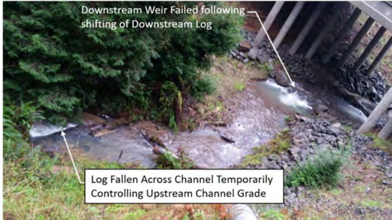
FIGURE 5-2. THE DESIGN ELEVATION AND DROP OVER THE DOWNSTREAM WEIR WAS BASED ON THE DOWNSTREAM CHANNEL BED ELEVATION CONTROLLED BY RECENTLY FALLEN LOG WITHIN THE CHANNEL BED, WHICH SUBSEQUENTLY SHIFTED, CAUSING THE BED TO DROP AND THE BOULDER WEIR TO FAIL.
