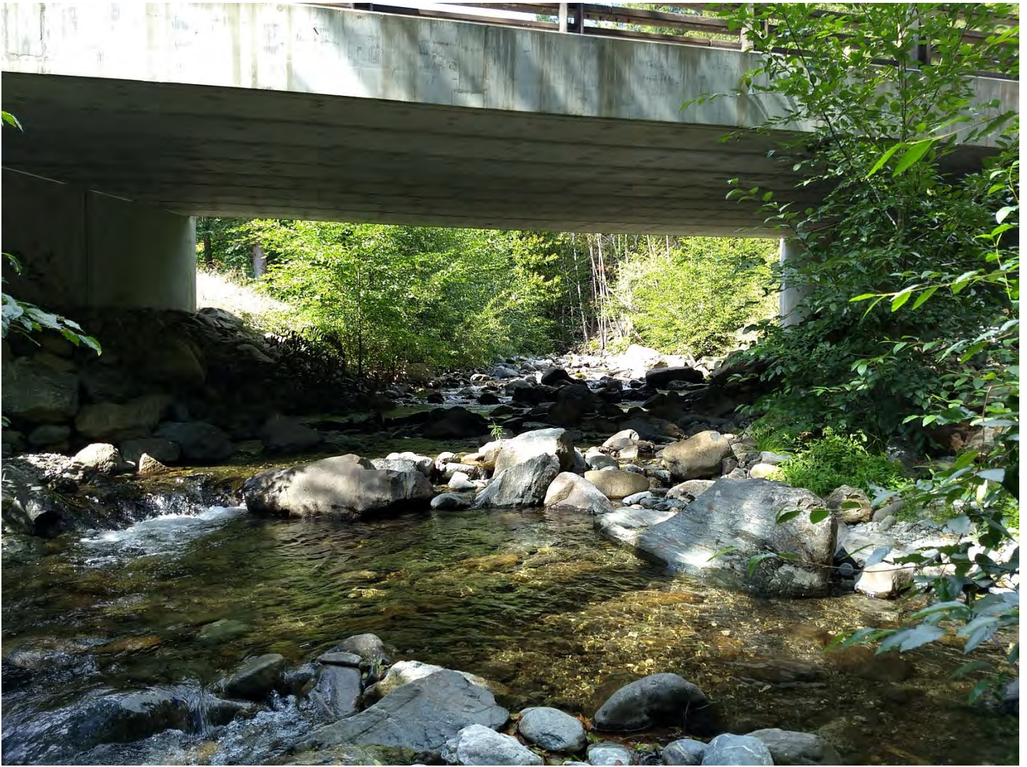
Figure 6. Channel and bridge looking upstream. Photo by M. Lang on 9/19/2019.
