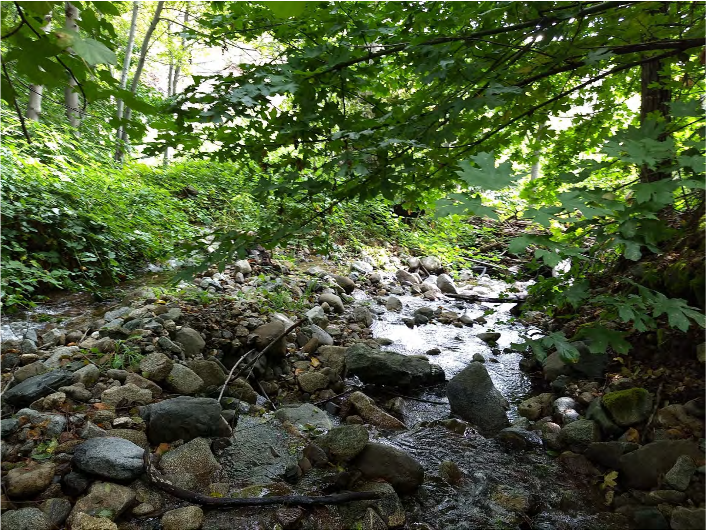
Figure 2. Channel downstream of the bridge looking downstream at the section with backwater deposits. There is a water diversion on the left channel that had been reworked to maintain its flow and elevation. The main channel is on the right. Photo by M. Lang on 9/19/2019.
