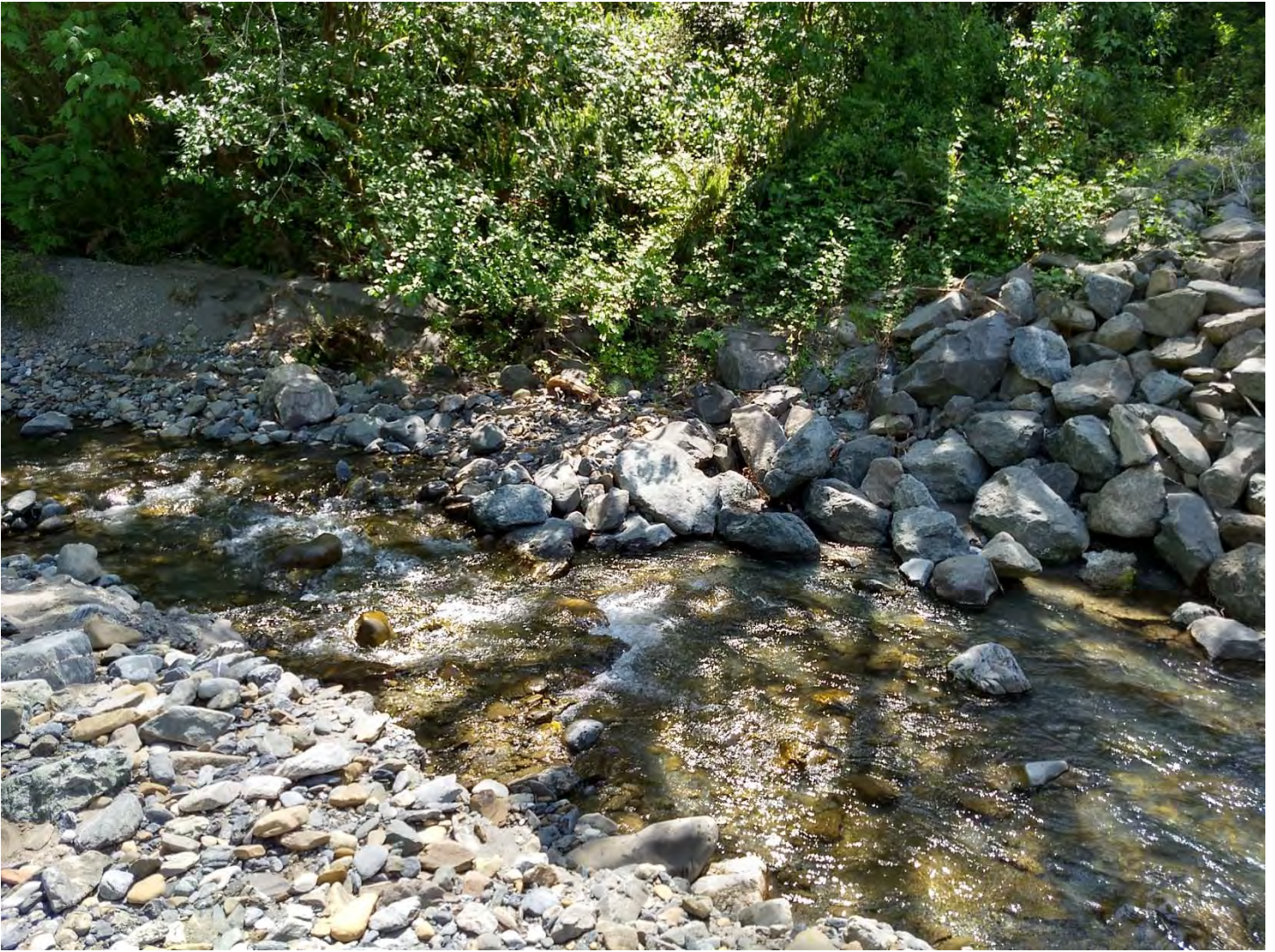
Figure 6. Missing/eroded rock weir grade control at upstream end of project site. Fish passage conditions are not compromised by the missing rock weirs.
