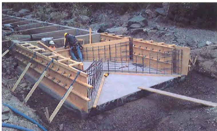
FIGURE 4-2. DOWNSTREAM FISHWAY EXTENSION UNDER CONSTRUCTION IN AUGUST, 2013.
