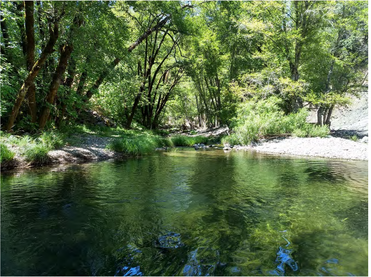
Figure 7. The outlet pool tailwater control looking downstream from the culvert outlet. Photo M. Lang on July 17, 2019.
