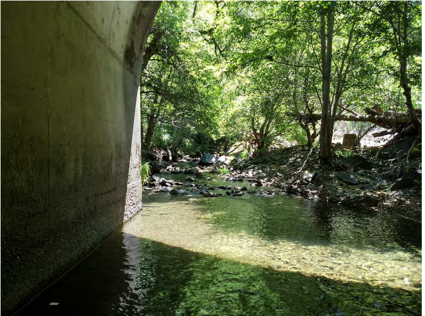
Figure 1. Looking upstream from the culvert inlet. Substrate in the channel is coarser here suggesting that the channel constriction due to a culvert width less than active channel width creates locally higher velocity than the natural channel. Photo M. Lang on July 17, 2019.
