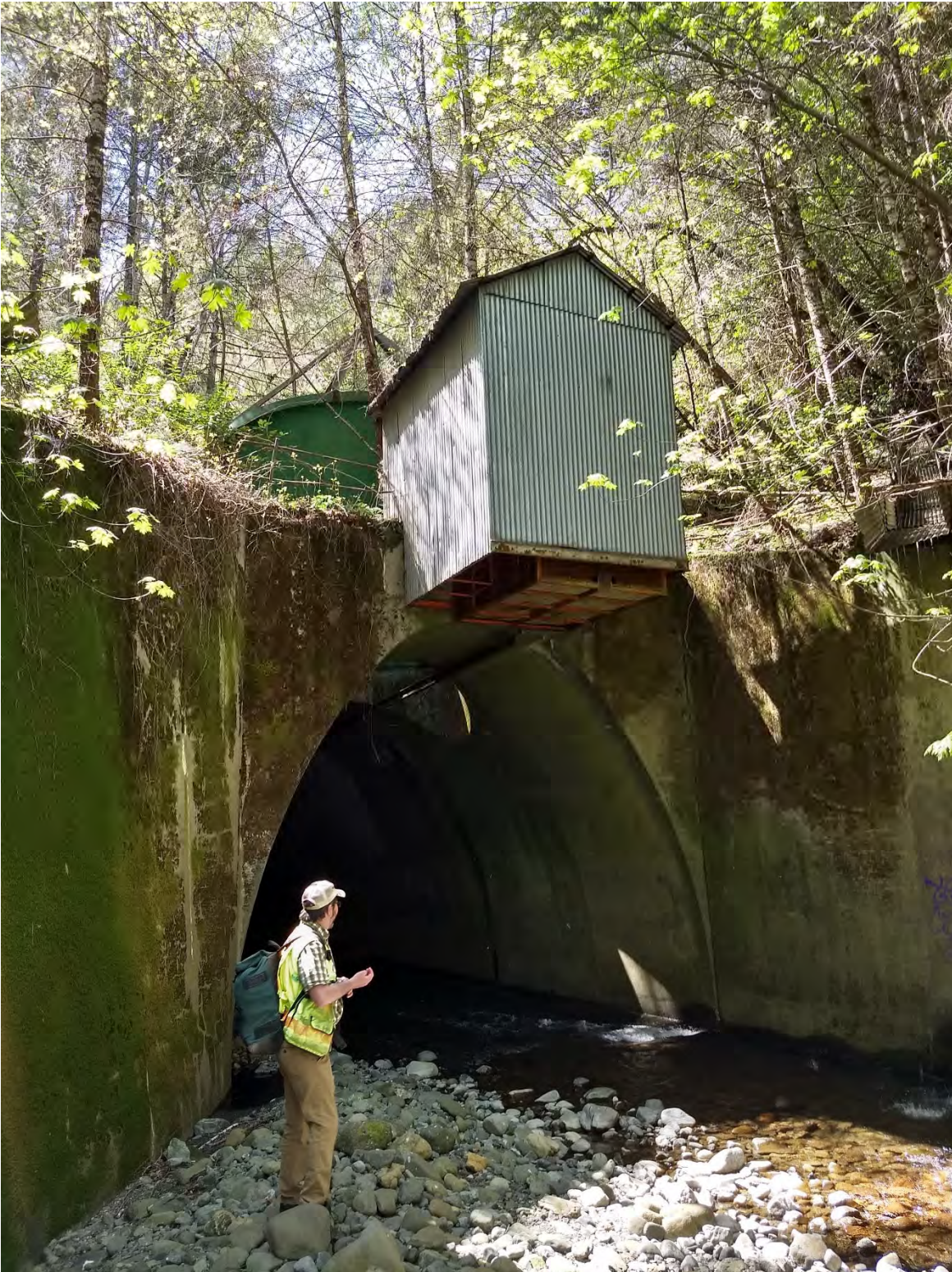
Figure 2. Cedar Creek culvert inlet. Photo taken by M. Lang April 15, 2021.
