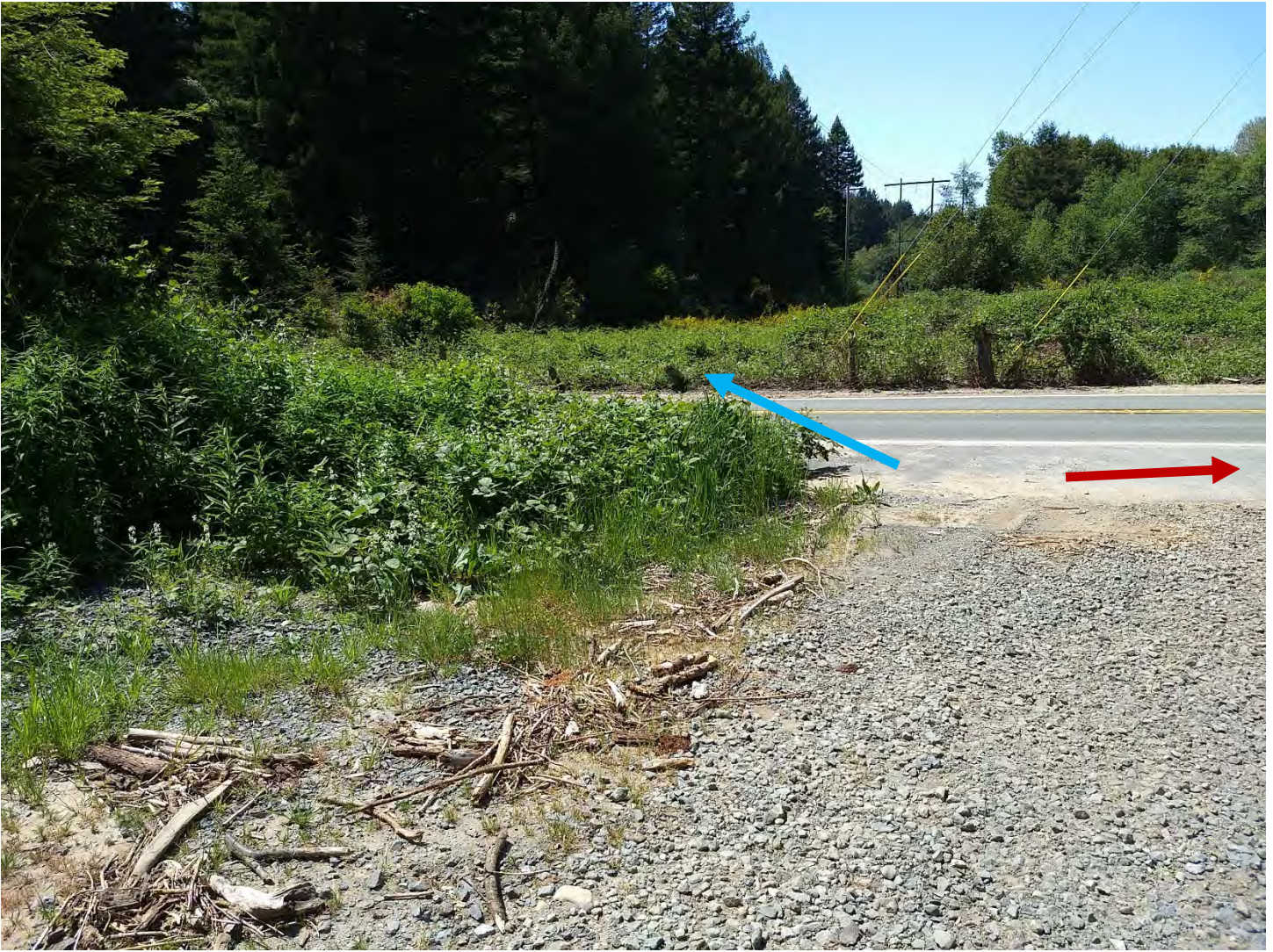
Figure 4. Intersection of Green Diamond access road and DN 197. Water along the road has deposited wood from the channel. Water that leaves the channel flows to the left on DN 197 (blue arrow); Sultan Creek is to the right (red arrow).
