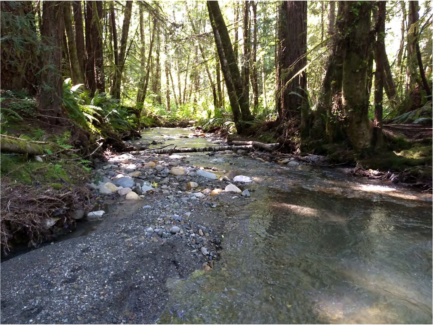
Figure 6. Downstream channel looking downstream from culvert outlet.
