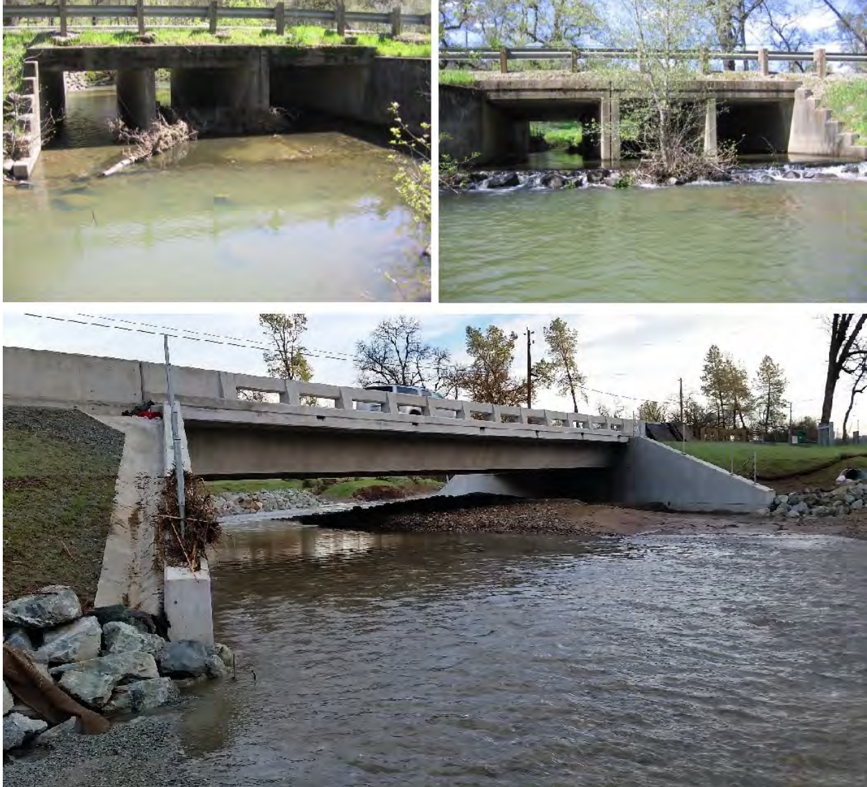
FIGURE 11-1. YANK (LEMM) CREEK CROSSING BEFORE THE BRIDGE CONSTRUCTION (TOP) AND LOOKING DOWNSTREAM AT THE REPLACEMENT BRIDGE IN 2015 (BOTTOM). THE TOP, LEFT PHOTO IS LOOKING DOWNSTREAM AT THE CROSSING AND THE TOP, RIGHT PHOTO IS LOOKING UPSTREAM SHOWING THE PERCHED APRON. NOTE THE HIGH WATER MARK DEBRIS ON THE INLET, LEFT WINGWALL. PHOTOS PROVIDED BY M. MOLINAR, CALTRANS.
