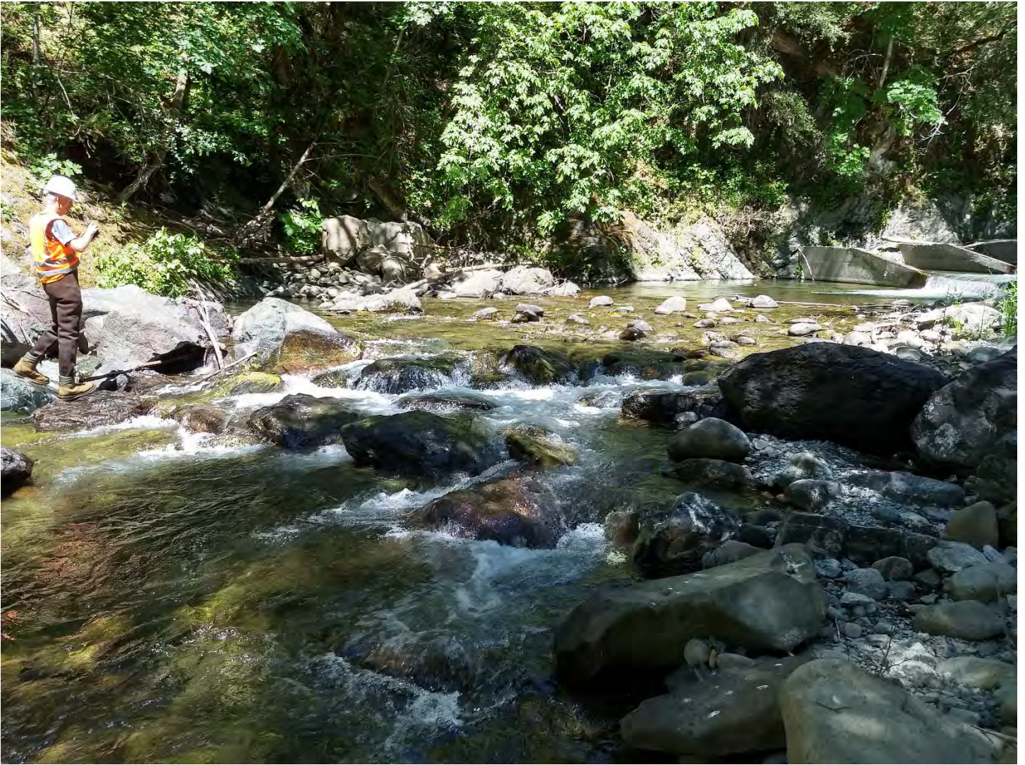
Figure 6. Looking upstream from the rock weir locations. In the foreground, the most downstream of the two rock weirs is somewhat intact. The most upstream rock weir is no longer present but its bank rocks are still present. The missing rock weir creates a larger drop height at the last fishway weir (~1.25 ft compared to 0.5 ft at most of the other weirs). Photo taken June 3, 2021.
