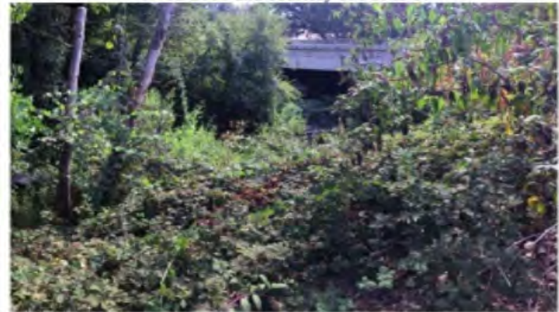
Bridge Inlet Post-Remediation. Photo taken on 09/12/2018 and courtesy of PSMFC.
