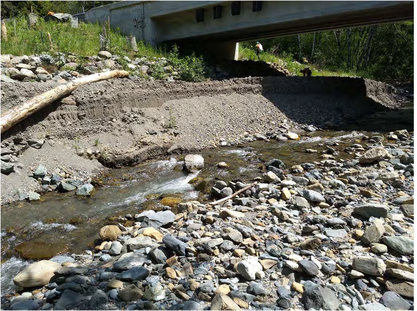
Figure 4. Right bank sediment deposit looking US through project site – closer view.
