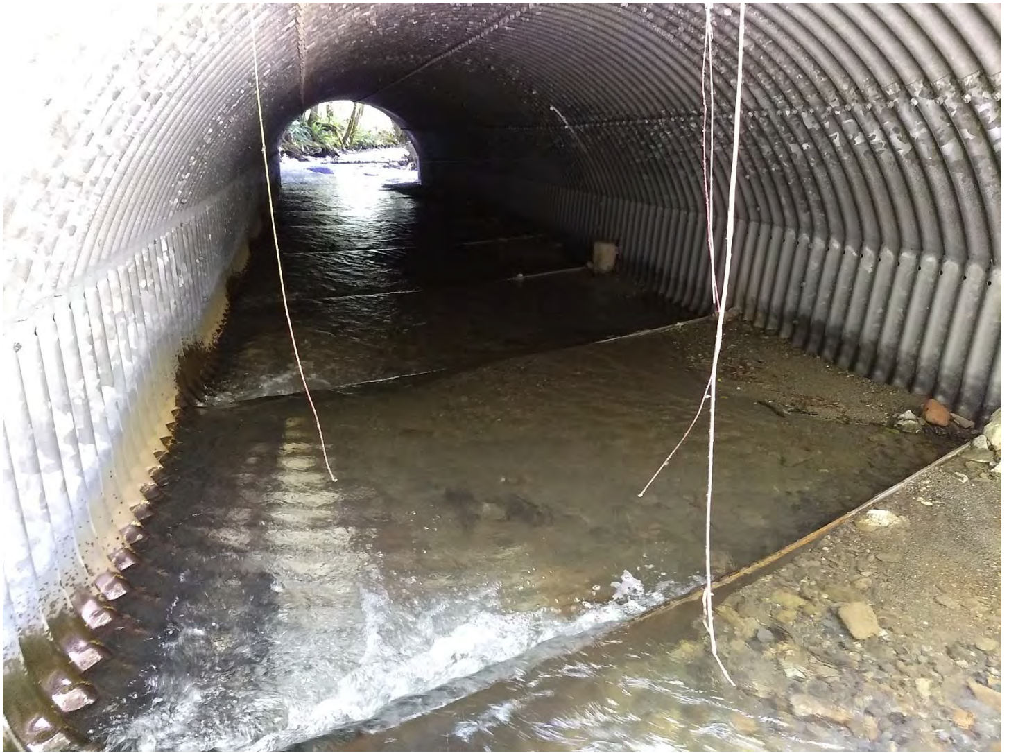
Figure 3. Culvert barrel looking downstream from the inlet.
