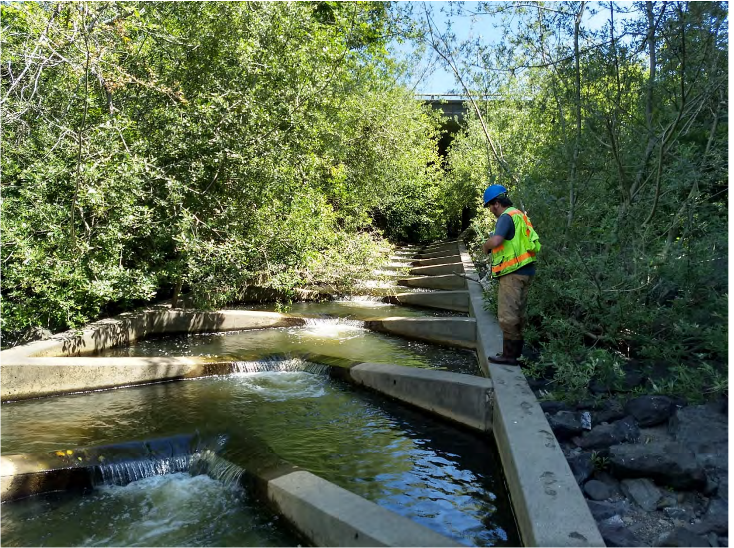
Figure 4. Hall Creek fish ladder looking upstream to the inlet transition under the HUM299 bridge. Photo taken by M. Lang June 6, 2020.
