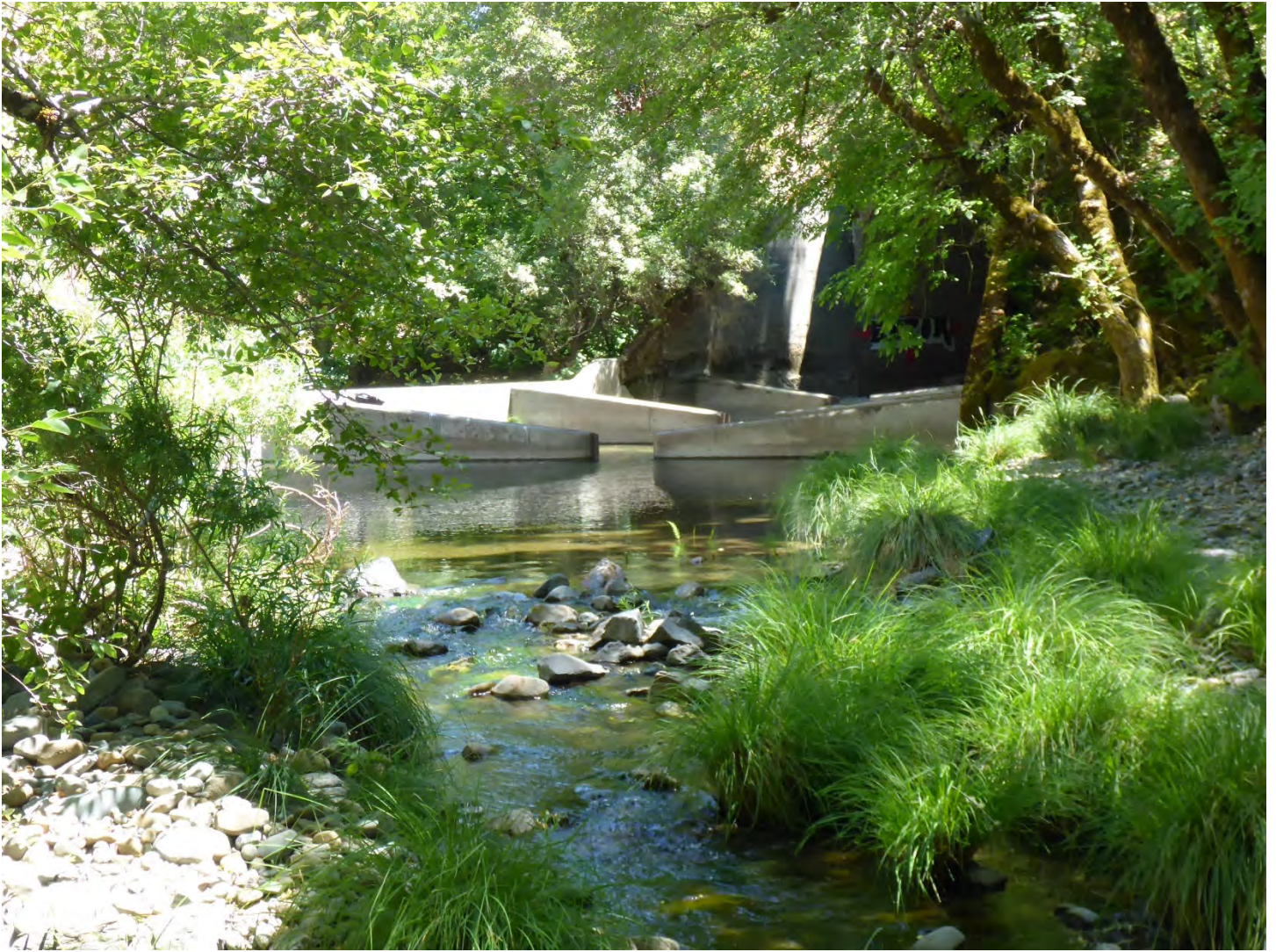
Figure 8. Outlet weirs looking upstream from the outlet pool tailwater control. Photo M. Love on July 17, 2019.
