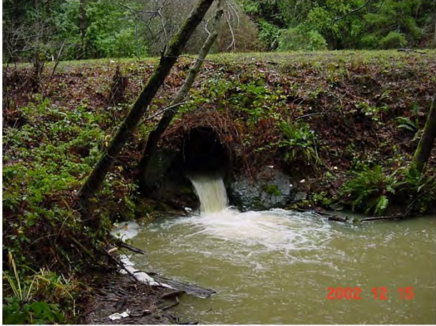
Culvert Outlet Pre-Treatment. Photo taken on 12/15/2002 and taken by HSU.
