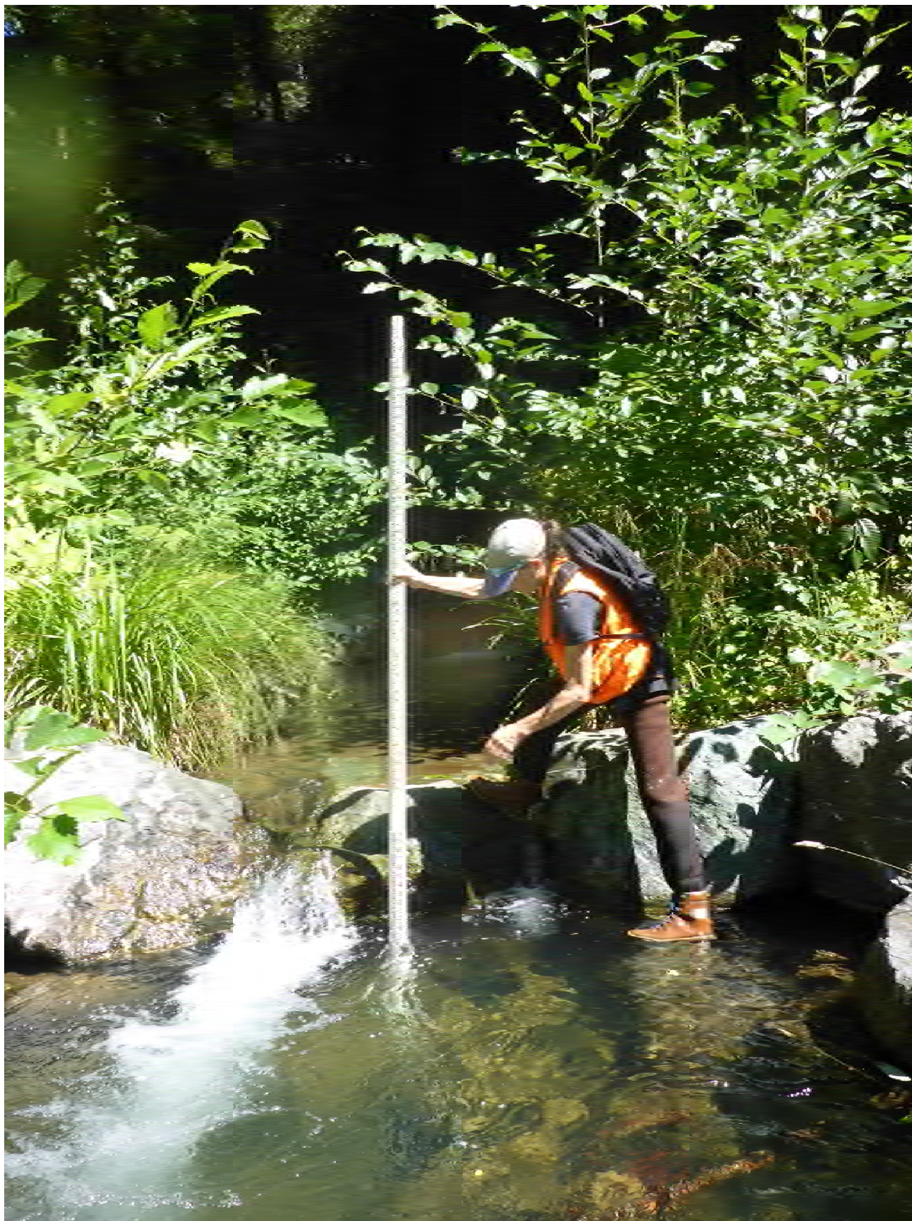
Figure 3. Upstream rock weir with deep plunge pool exposing foundation rock. Photo by Michael Love on 7/17/2019.
