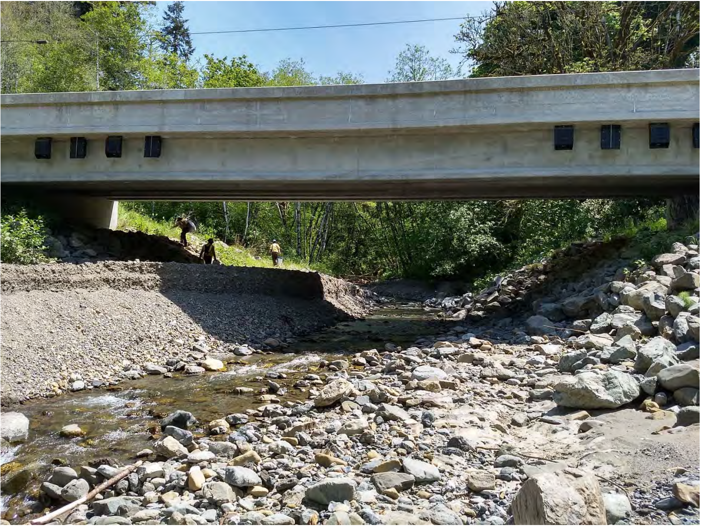
Figure 3. Right bank sediment deposit looking US through project site.
