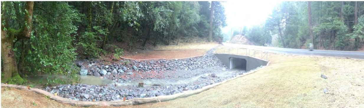
Culvert Inlet Post-Treatment. Photo taken on 01/09/2018 and courtesy of Caltrans.
