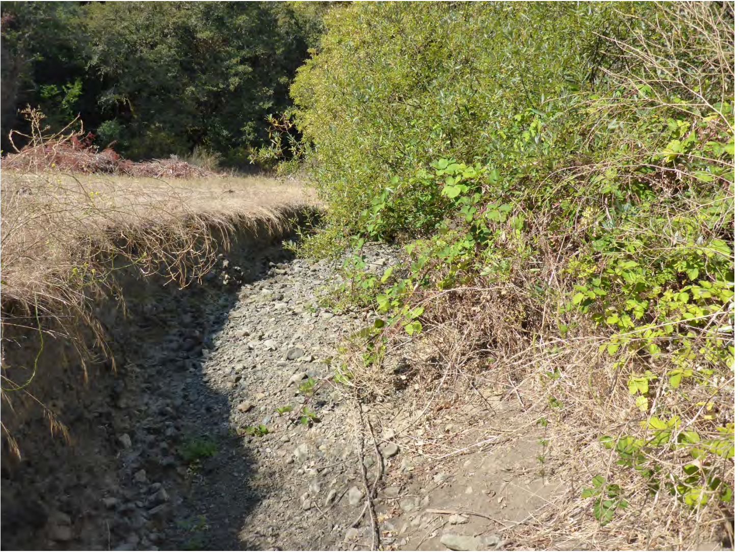
Figure 3. Upstream erosion on right bank, view is looking upstream and new bridge is downstream. Photo by Michael Love on 9/12/2019.
