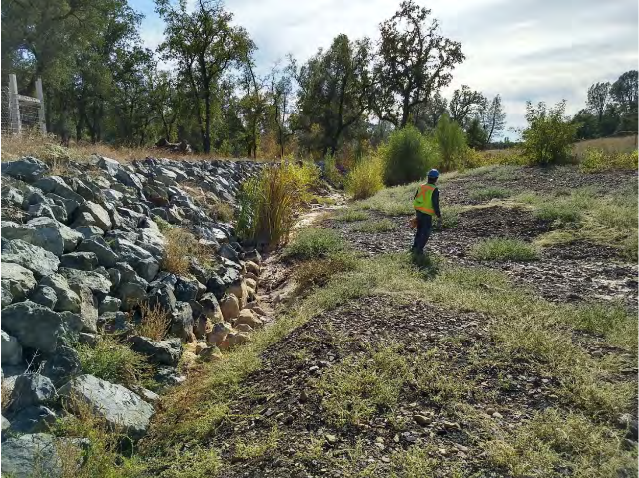
Figure 2. Lemm/Yank Creek Highway 299 bridge looking downstream at the downstream channel just after the bridge. This section makes a sharp right turn along the armored embankment into a narrow, V-shaped channel for approximately 60 feet before the downstream channel widens and transitions to a natural channel shape with a mix of claystone bedrock sections and gravel. Photo taken October 4, 2019.
