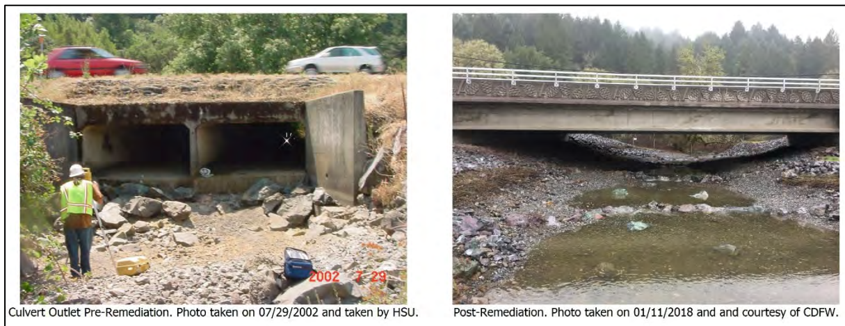
FIGURE 6-1. PRE AND POST PROJECT LOOKING UPSTREAM AT CROSSING.
